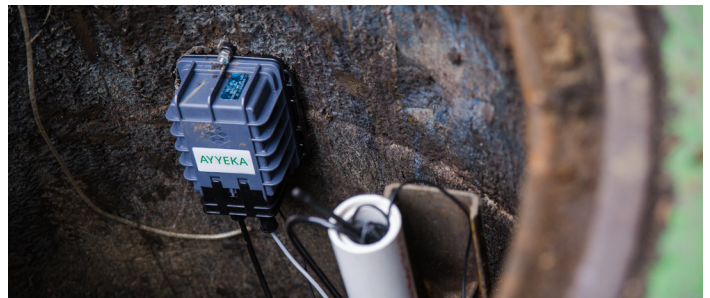
Installation of Wavelet Sewer Overflow Kit in San Francisco, CA.
