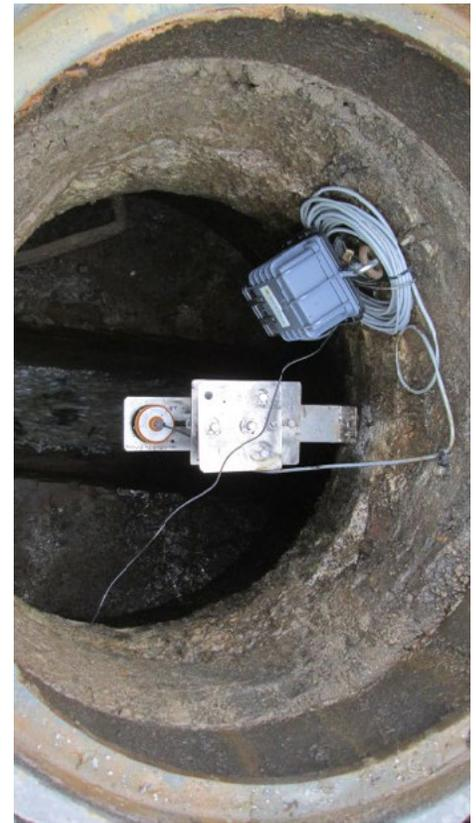
Image 4: Field installation of Ayyeka Wavelet Ultrasonic CSO Kit for sewer level data acquisition in Cincinnati.
